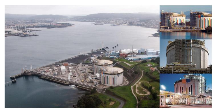
Storage tanks are a significant part of any LNG project cost. There are several basic designs including single containment (with an inner container made of 9% Ni steel able to withstand cryogenic temperatures), double containment (in which an outer container made of concrete provides a second barrier to contain the leaks), and full containment tanks (in which an outer layer made of pre-stressed concrete completely encases the tank to provide a second containment system.)
